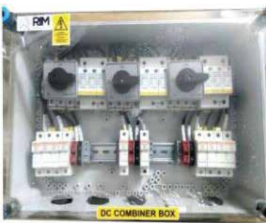
String Combiner box with Five inputs with String fuses and Three outputs with three isolators and three surge protection devices
